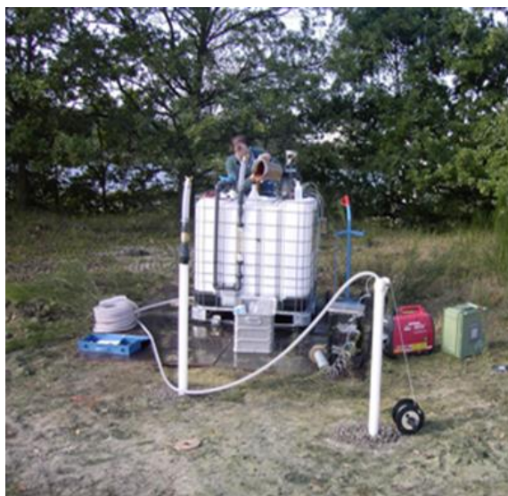
Figure 12 Injection of substrate via permanent vertical wells to create a reactive zone.
