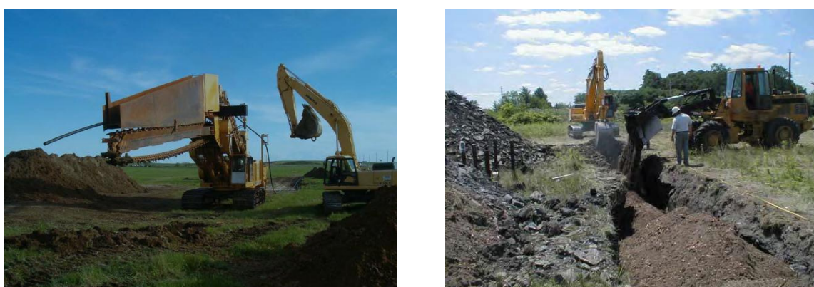
Figure 14: Implementation of biobarriers via continuous trenching (left) and refill of a trench (right).
