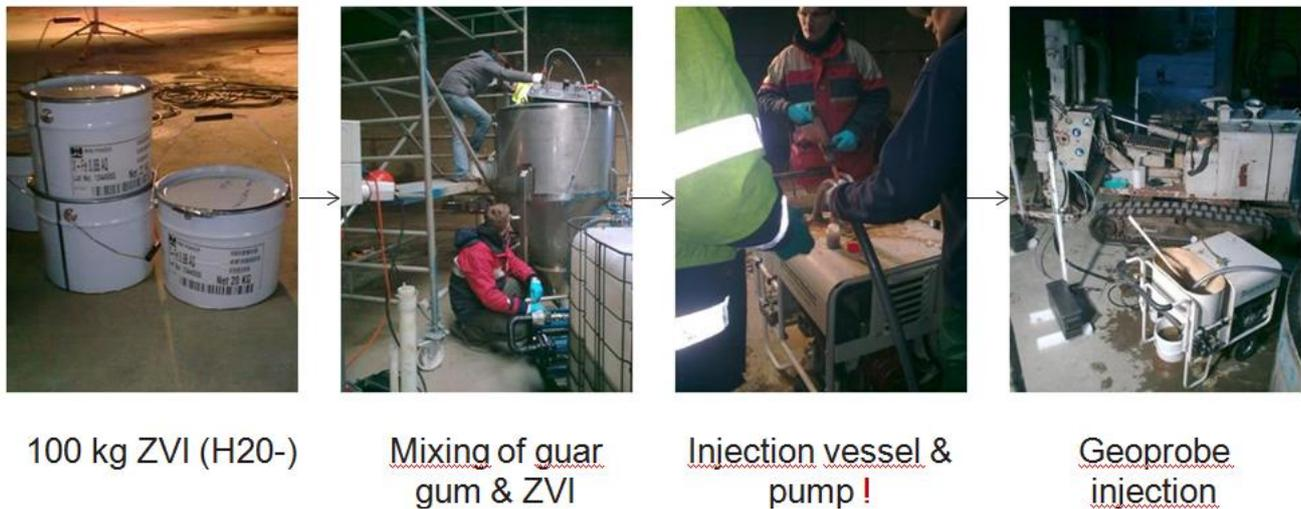
Figure 34 Preparation and immediate use of the ZVI-suspension as performed within AQUAREHAB for a small pilot test (injection of 100 kg mZVI, 1.6 m<sup>3</sup> ZVI suspension).
