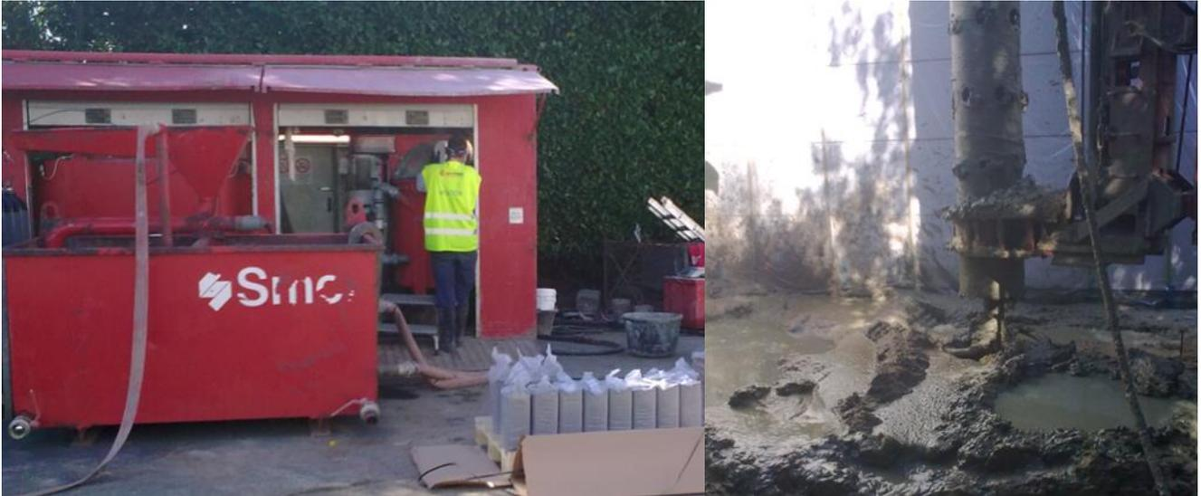
**Figure 36 Large scale preparation of mZVI-slurry for a soil mixing application using an existing device designed for bentonite mixing.**
