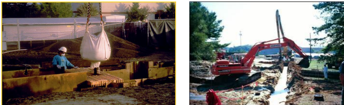
Figure 6: Implementation of ZVI-barriers (SOURCE: ETI)
