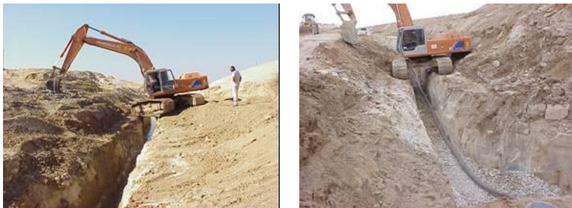
Figure 5. Pictures showing the trenches dug perpendicular to the main flow direction in fractures to focus groundwater flow technology.
