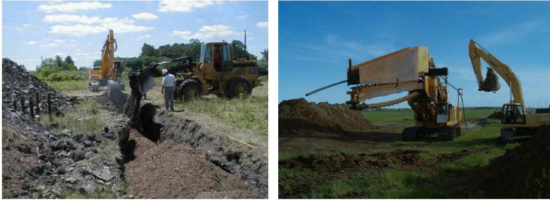
Figure 4: Implementation of biobarriers (Left) continuous trencher, (Right)
